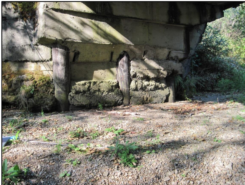
Photo 4: Looking west at Bent 2
