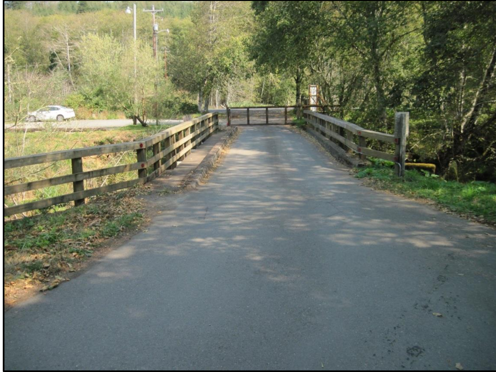
Photo 1: Looking east at the South Beach Road Bridge
