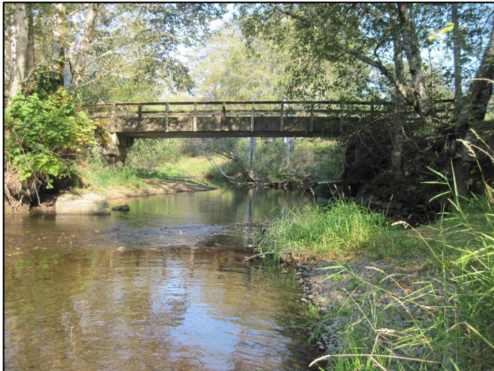
Photo 2: Looking downstream at the South Beach Road Bridge.
